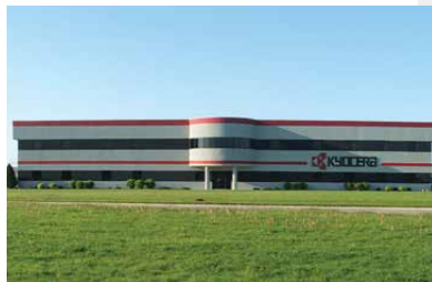
Ohio Facility (USA)
