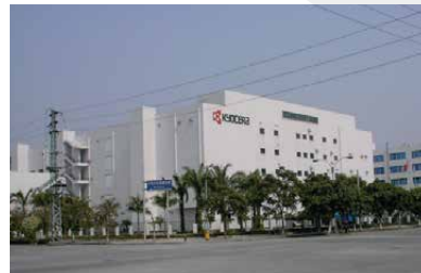
Silong Facility (CHINA)
