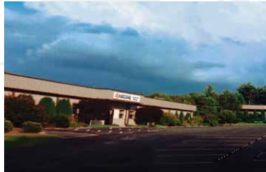
North Carolina Facility (USA)
