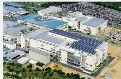
Yokaichi Facility (JAPAN)
